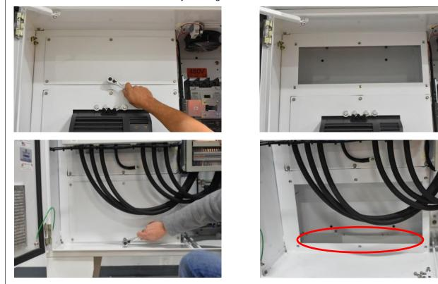
4a) To access top exhaust screen, loosen external screws located on the front and back of Enclosure and lift off the top hood.
